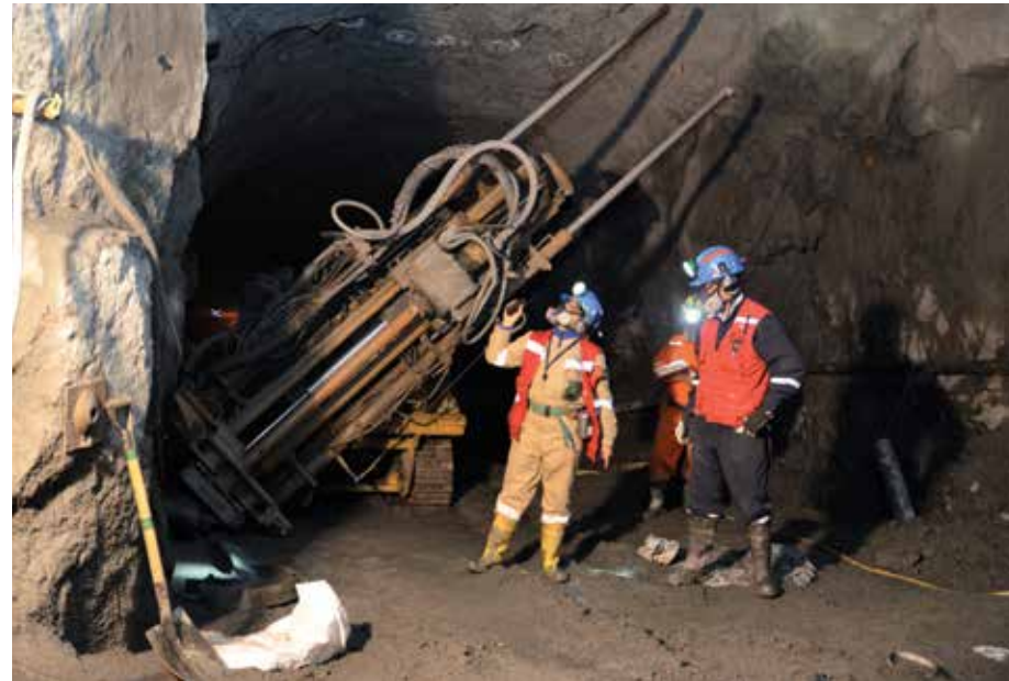
Underground Drilling Operations, Candelaria
