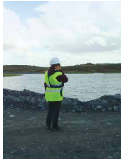
Tailings Management Facility, Neves-Corvo
