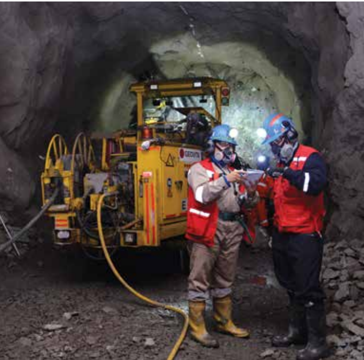
Underground Operations, Candelaria
