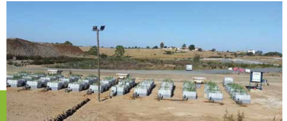
View of the passive water treatment trials
