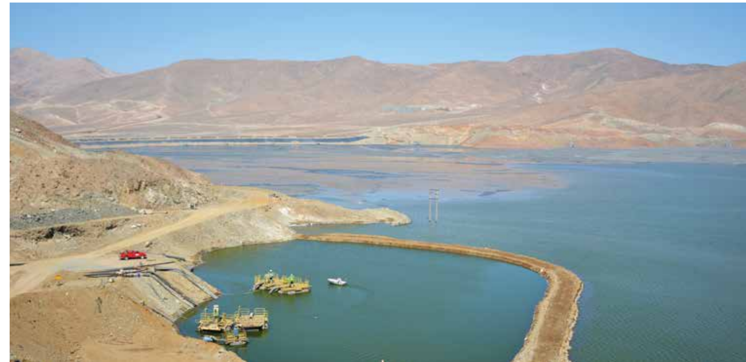
Mine Water Recovery System and Tailings Storage, Candelaria
