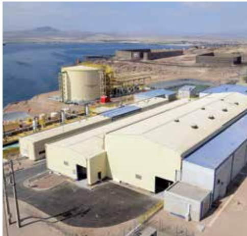
Candelaria Desalination Plant, Punta Padrones Port Facility
