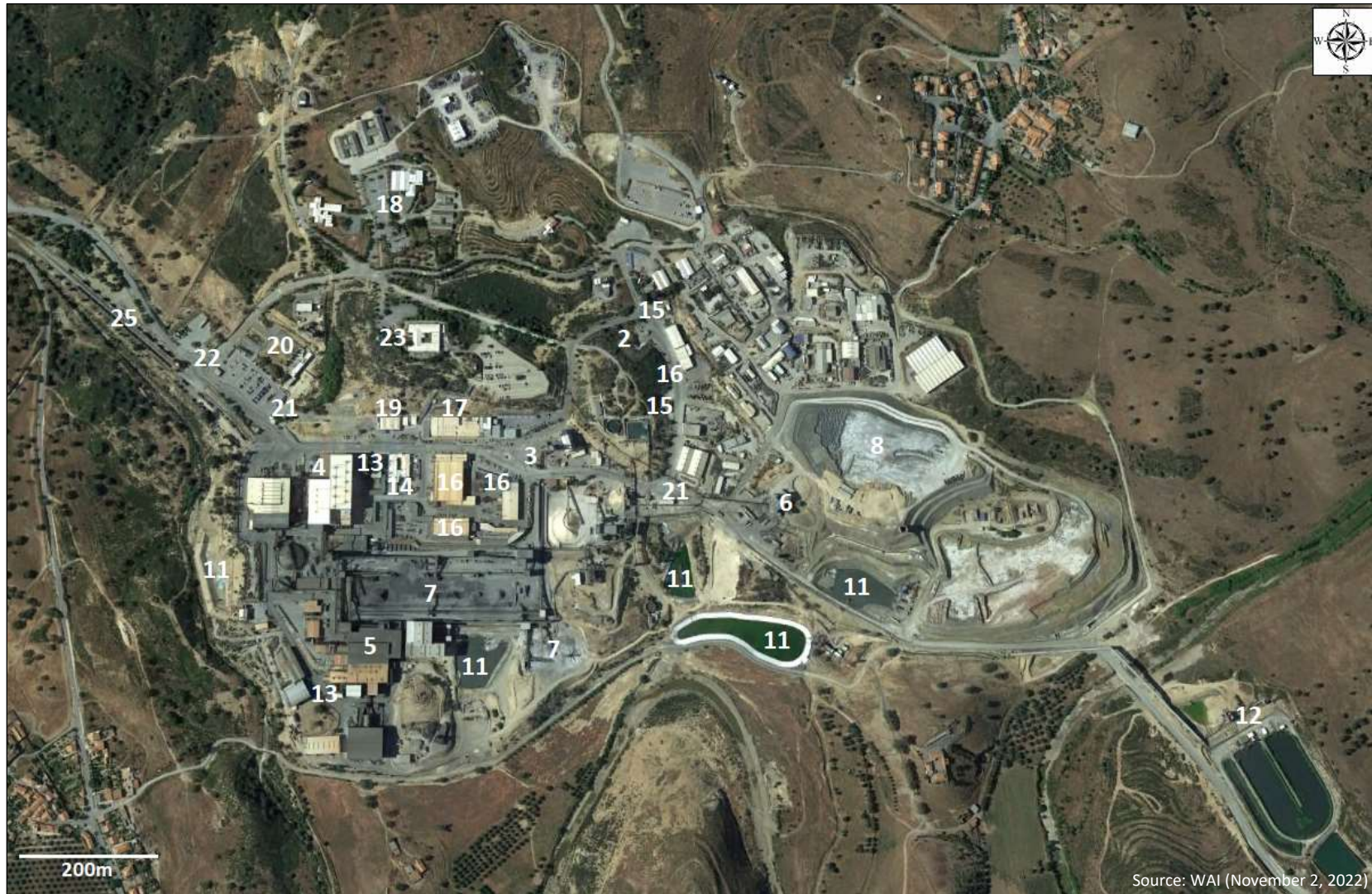
Figure 18.2: Neves-Corvo Mine Infrastructure (Inset of Figure 18.1)
