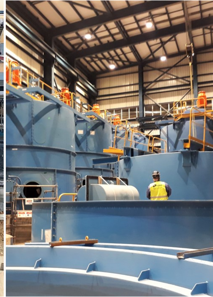
Flotation Cell Installation
