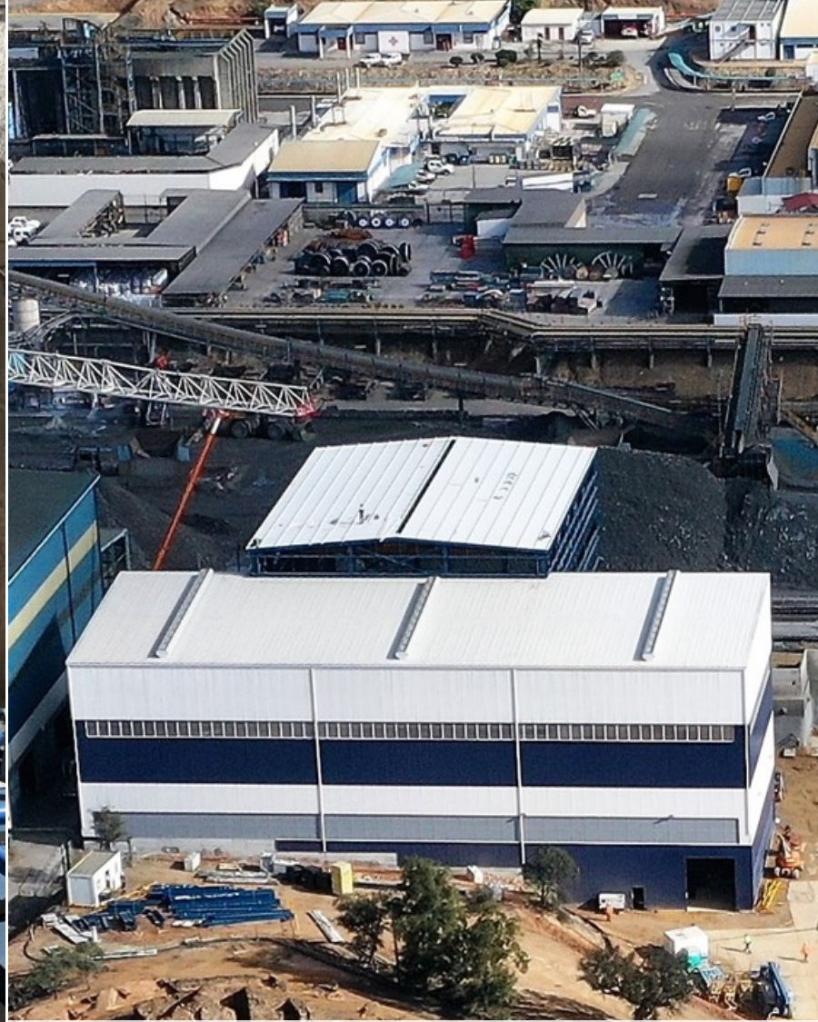
Flotation and Filtration Buildings
