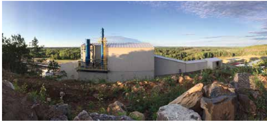
Eagle Mine – Humboldt Mill Concentrator Building at Sunrise
