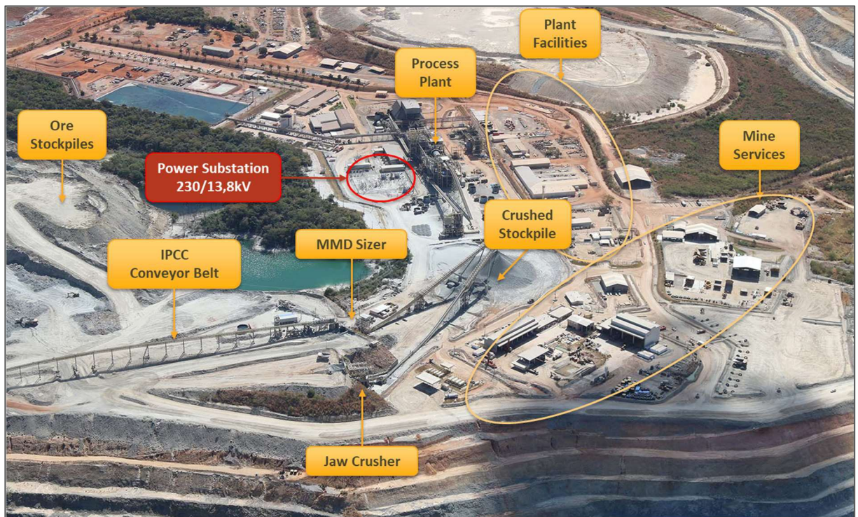
Figure 16-1: Overview of Chapada Process Plant Facilities
