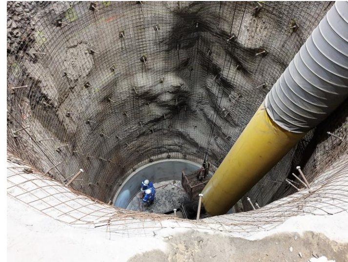
Silo G lining
