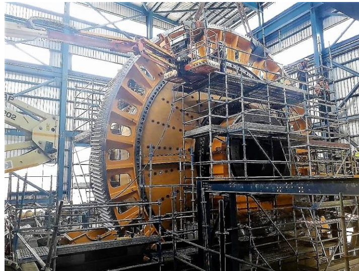
SAG mill gear ring installed
