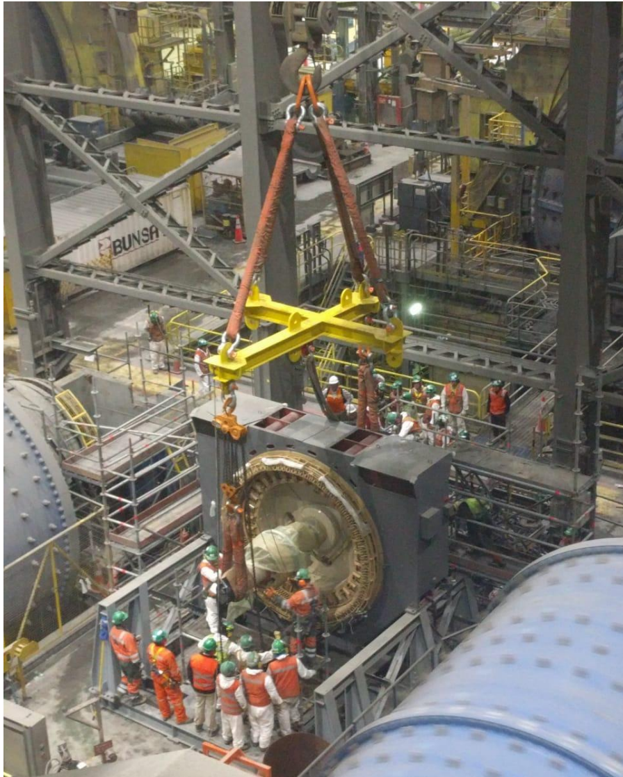
Candelaria Ball Mill 2 motor replacement
