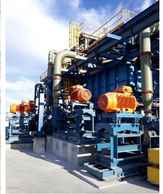
Cyclones area piping installation
