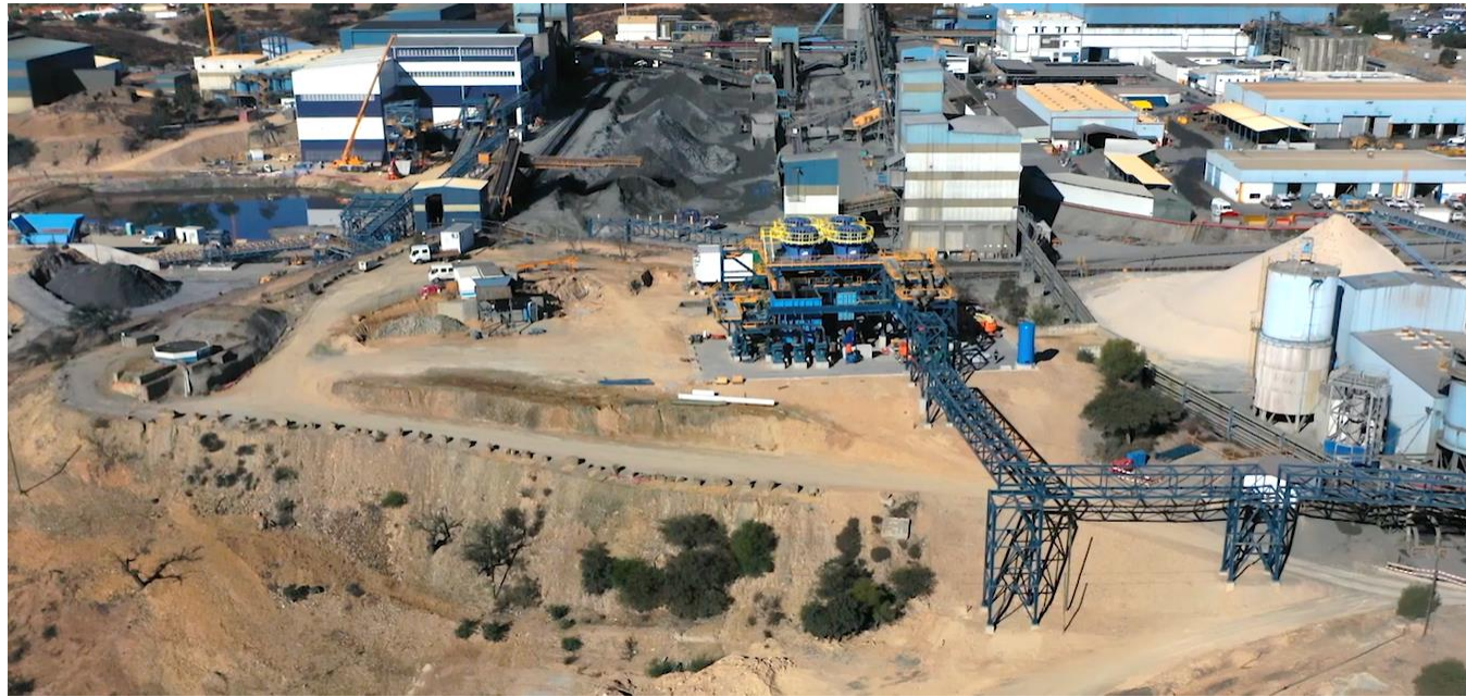
Cyclone station in center, new mill building in background
