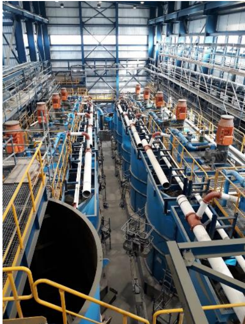
New flotation building piping installation
