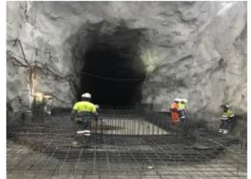
Silo 7 ground support complete
