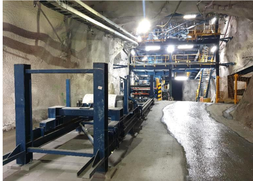
Installation of Transfer Station 3 ongoing
