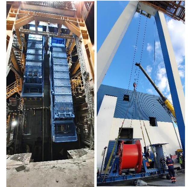
New skips and hoisting rope installed
