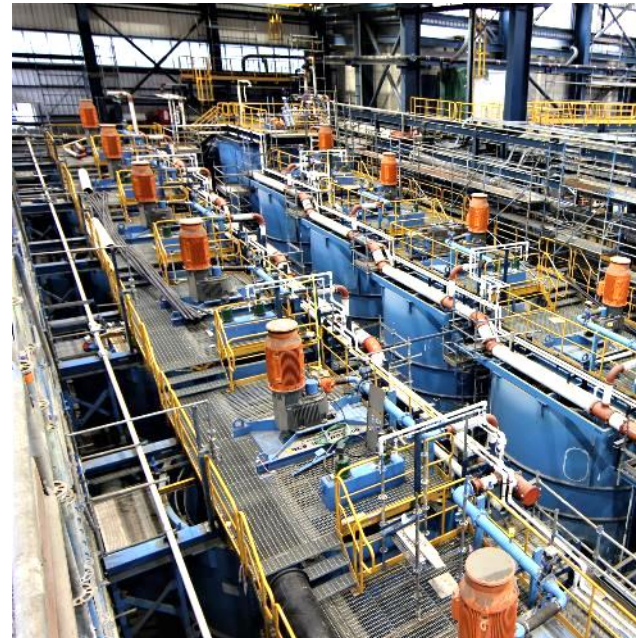
New flotation building piping installation – December 2020
