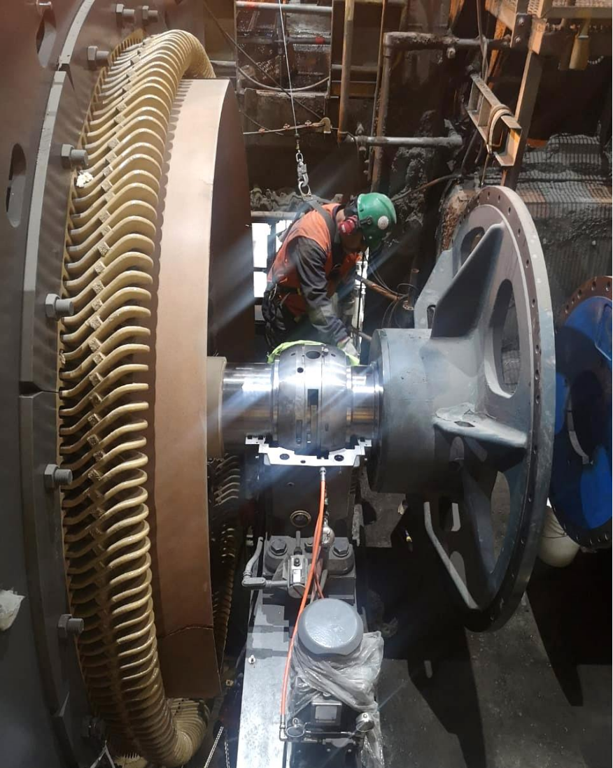
Candelaria mill ball third motor replacement during Q4/19
