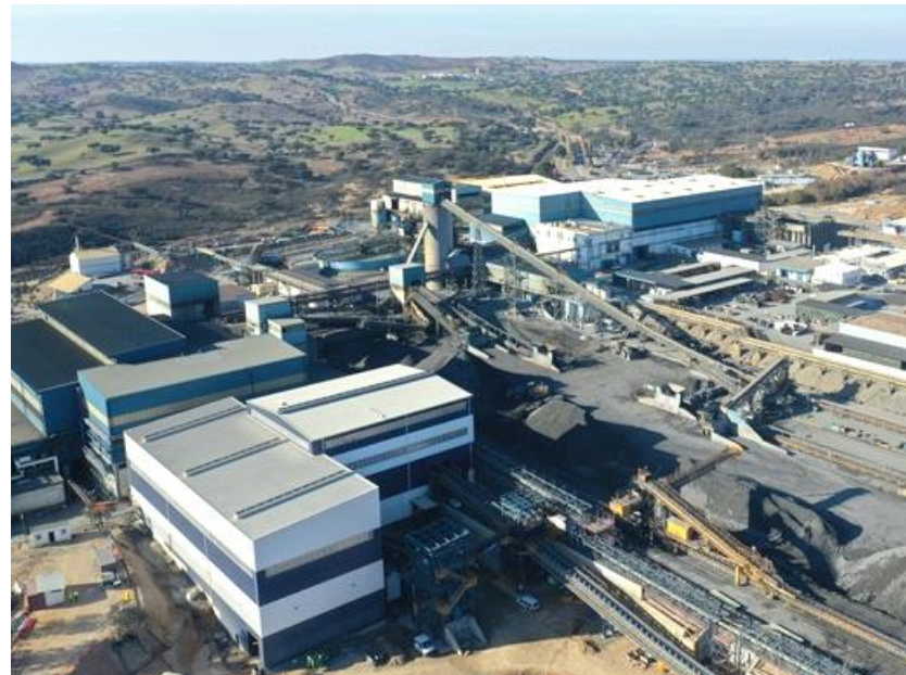
New ZEP mill and flotation buildings in foreground – January 2020
