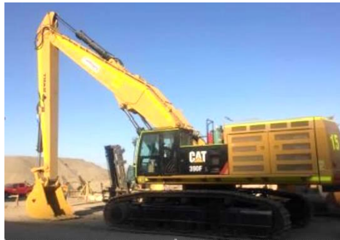
Last 390FL Excavator with long reach boom arrived in November 2019
