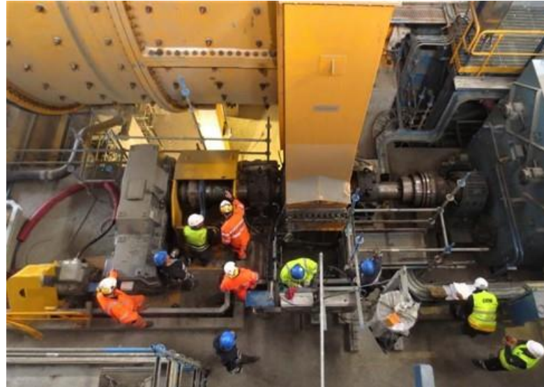
SAG mill commissioning work
