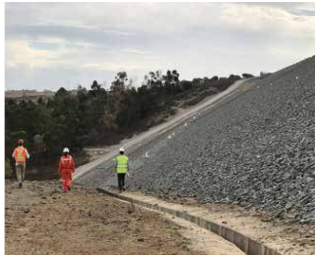
Neves-Corvo – Tailings Facility
