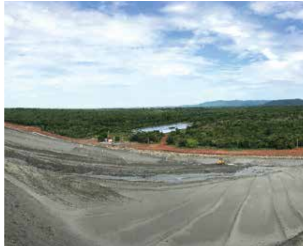
Chapada – Tailings Facility
