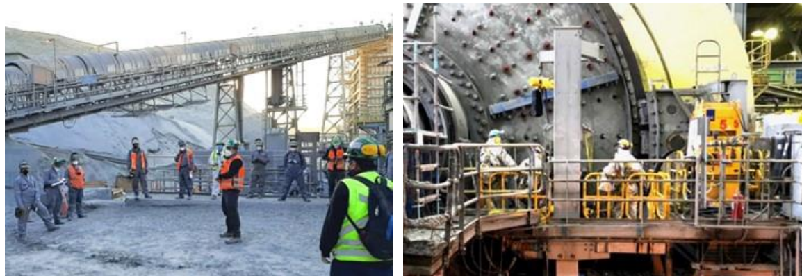
Crusher and mill maintenance – February 2021
