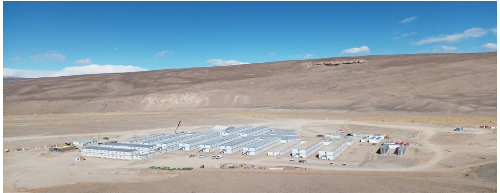
Josemaria Copper-Gold project camp construction, San Juan, Argentina – April 16, 2022
