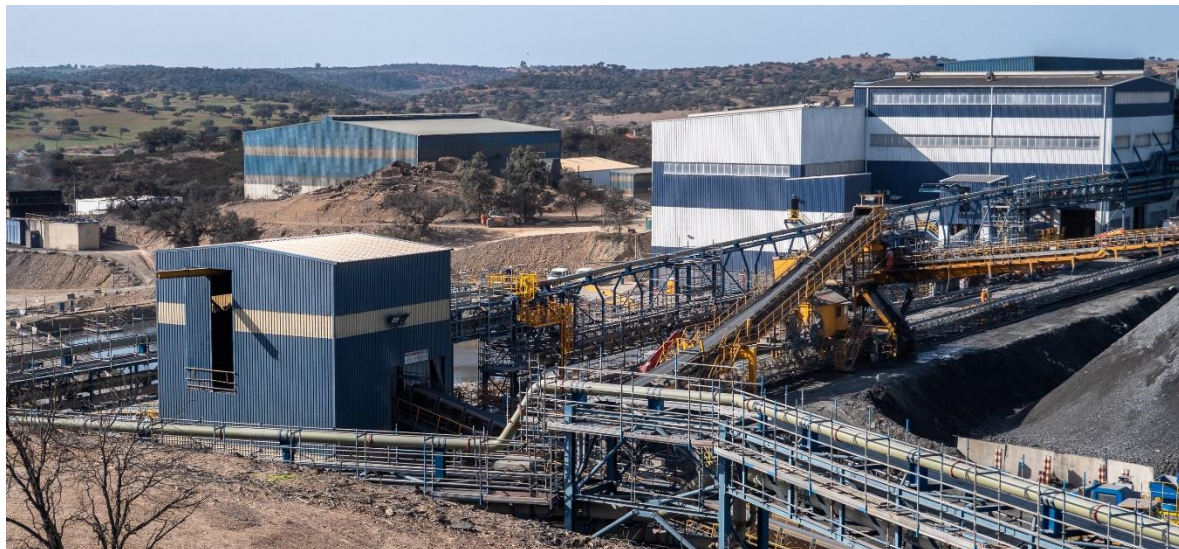
ZEP surface facilities – February 2022
