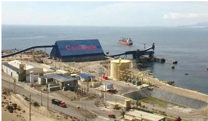
Candelaria Punta Padrones port and desalination plant
