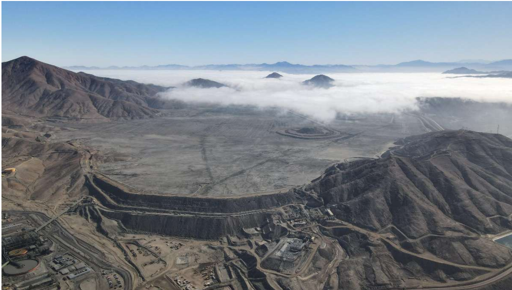
Figure 1: Candelaria Tailings Storage Facility
