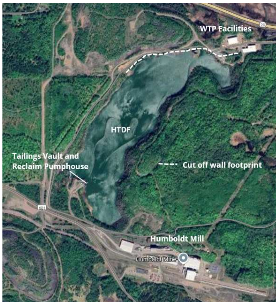
Figure 1: Humboldt Tailings Disposal Facility Actual Layout
