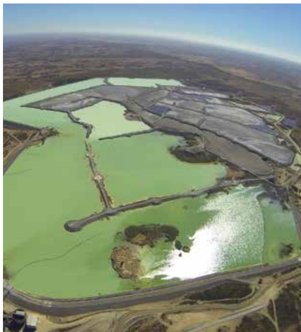
Tailings Facility, Neves-Corvo, Portugal
