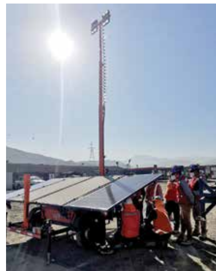
Solar Panels Installed, Candelaria, Chile
