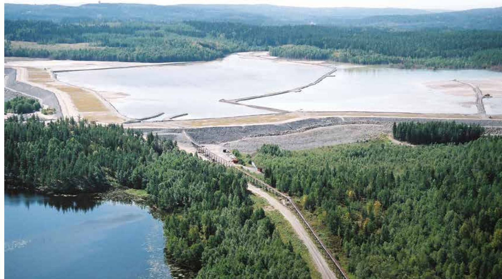
Tailings Facility, Zinkgruvan, Sweden
