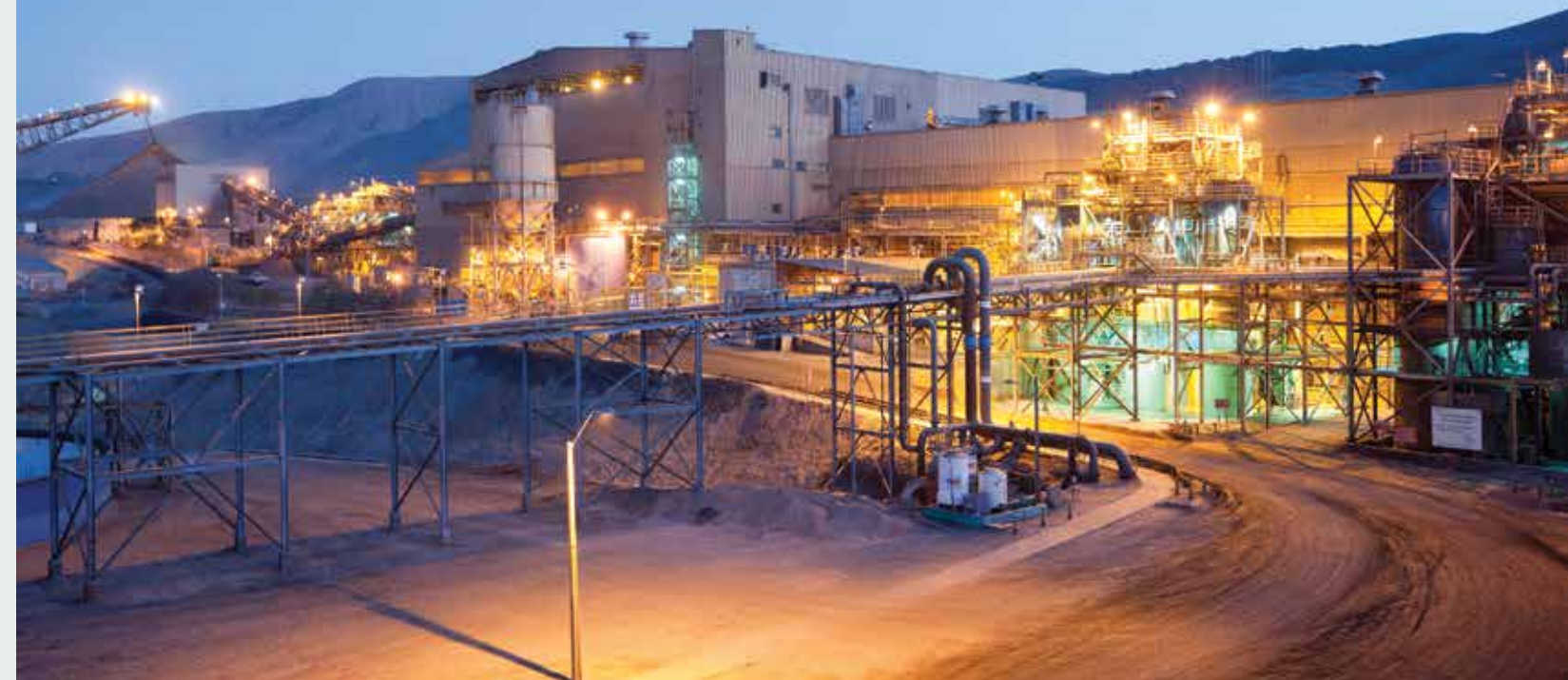
Mill Process Plant, Candelaria, Chile
