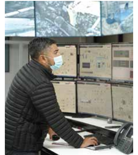
Processing Plant Control Room, Candelaria, Chile
