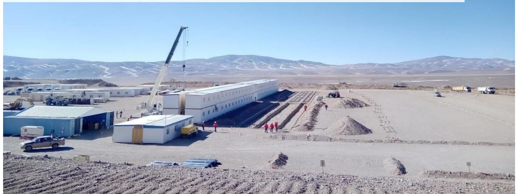
Construction on Josemaria Project Camp
